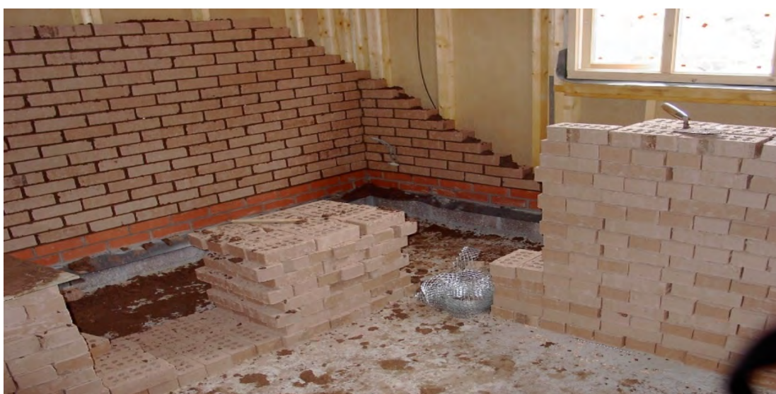
Fig. 22: Earth mortar in contemporary eco-house, Perthshire.
