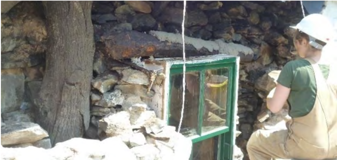
Fig. 8: Back face of inner leaf exposed during repairs at Moirlanich, with cruck leg having benefitted from the preserving effect of earth mortar drawing away moisture.
