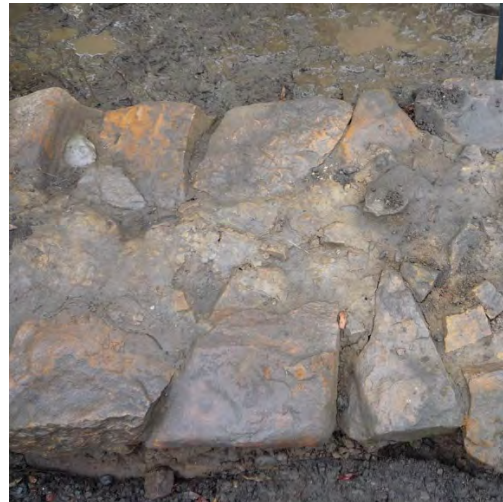
Fig. 14: Earth mortar, note no lime.
