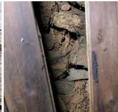
Fig. 20: Earth mortar concealed behind internal linings.
