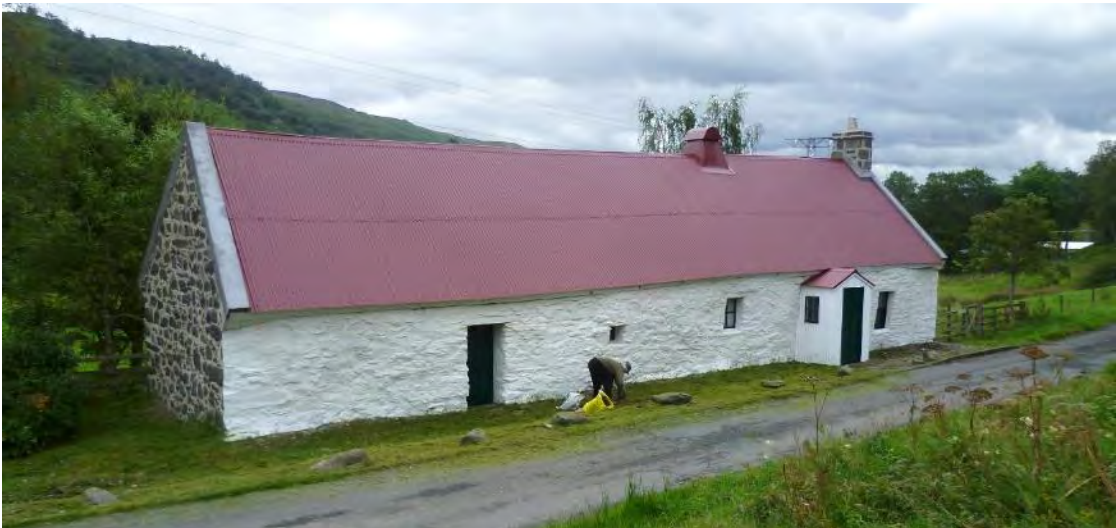
Fig. 7: Moirlanich Longhouse, weak earth mortared rubble with lime pointing & wash. The leaning section to the right of the porch is shown in repair below.
