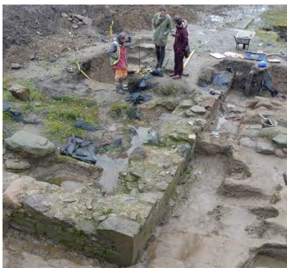
Fig. 15: Carmelite Friary, Perth, earth mortared wall bases, may have had lime mortared masonry above.
