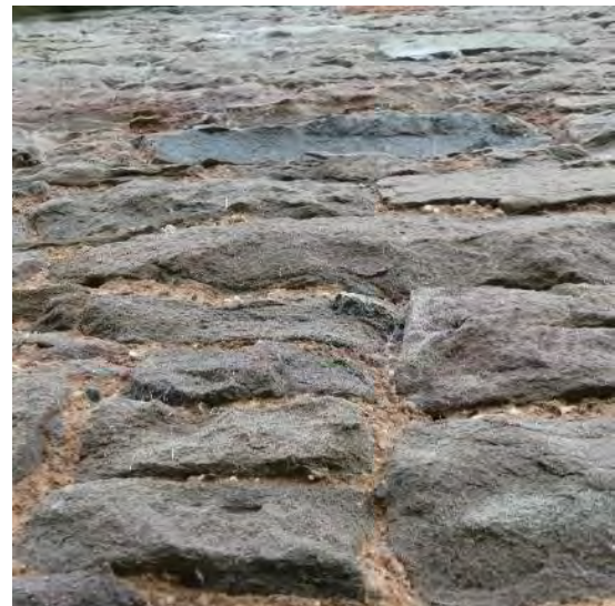
Fig. 11: Detail of earth-lime mortar.
