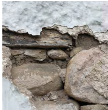
Fig. 19: Earth mortar concealed behind lime finishes.
