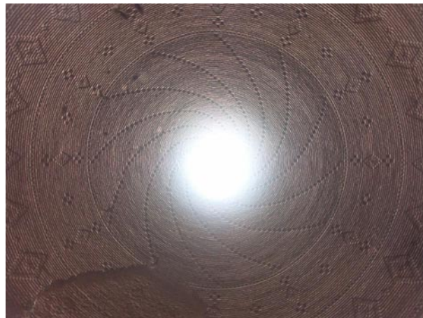
19. Interior of Dome, Moayedi, Kashan
