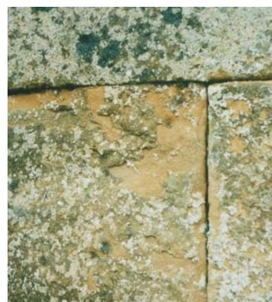
The existing lichen will be lightly sprayed with an approved biocide and left to die off. The dead lichen will then be removed with a dental steam machine, carefully worked over each surface and controlled to as not to over clean the stone.
