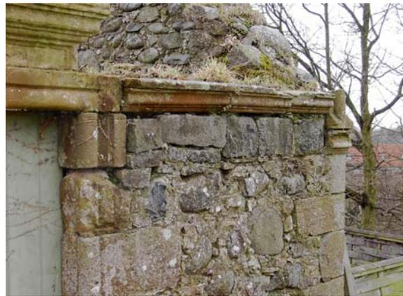
4.2.4 **Pediment Stones.** On the west wall, above the door, stands a corniced sandstone panel, with the inscription 'Rep'd 1831'. There is a similar stone on the east wall, over the central armorial panel. This stone has no inscription and is raised up on two small rectangular basalt blocks, the rest of the elevation being dressed sandstone. Both these stones have roughly hewn backs and are much more weathered than the others in their vicinity.
