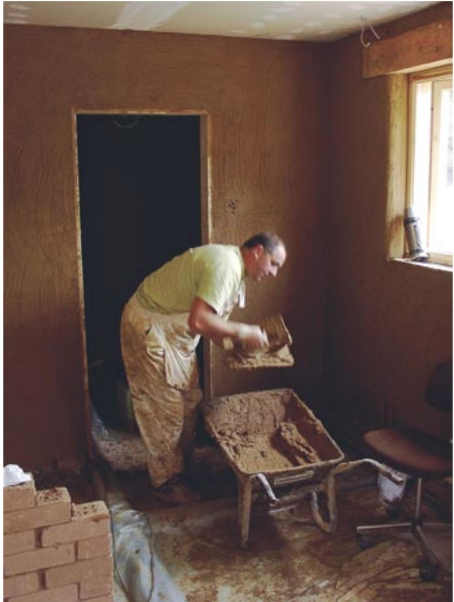
Timber frame building in reverse - frame and timber cladding on outside and heavy masonry as interior skin.
