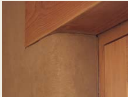
page 4 Clay plaster wall finish can be left natural or painted
