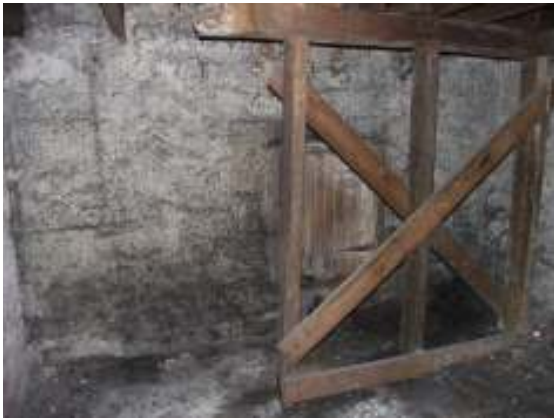
Fig 19: The Ground Floor room.
