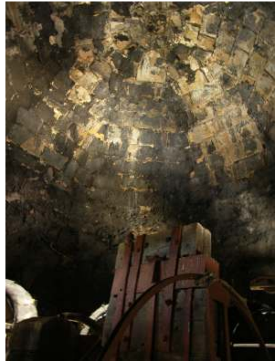
Fig 24: The belfry vaulted ceiling.
