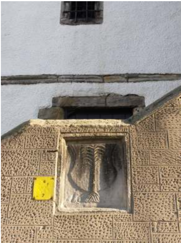
Fig 17: The 1617 armorial panel.
