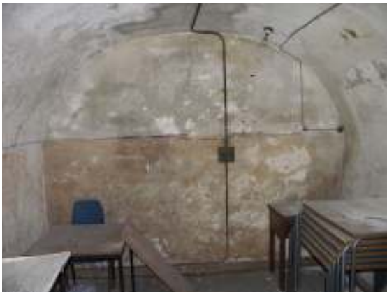
Fig 20: The First Floor room.
