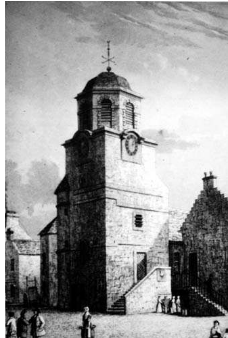
Fig 10: View, undated. This image shows the tower stripped of render, revealing coursed rubble.
