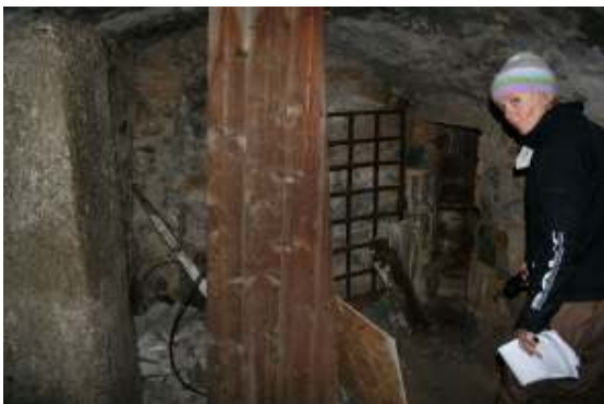
Fig 22: The Third Floor room.
