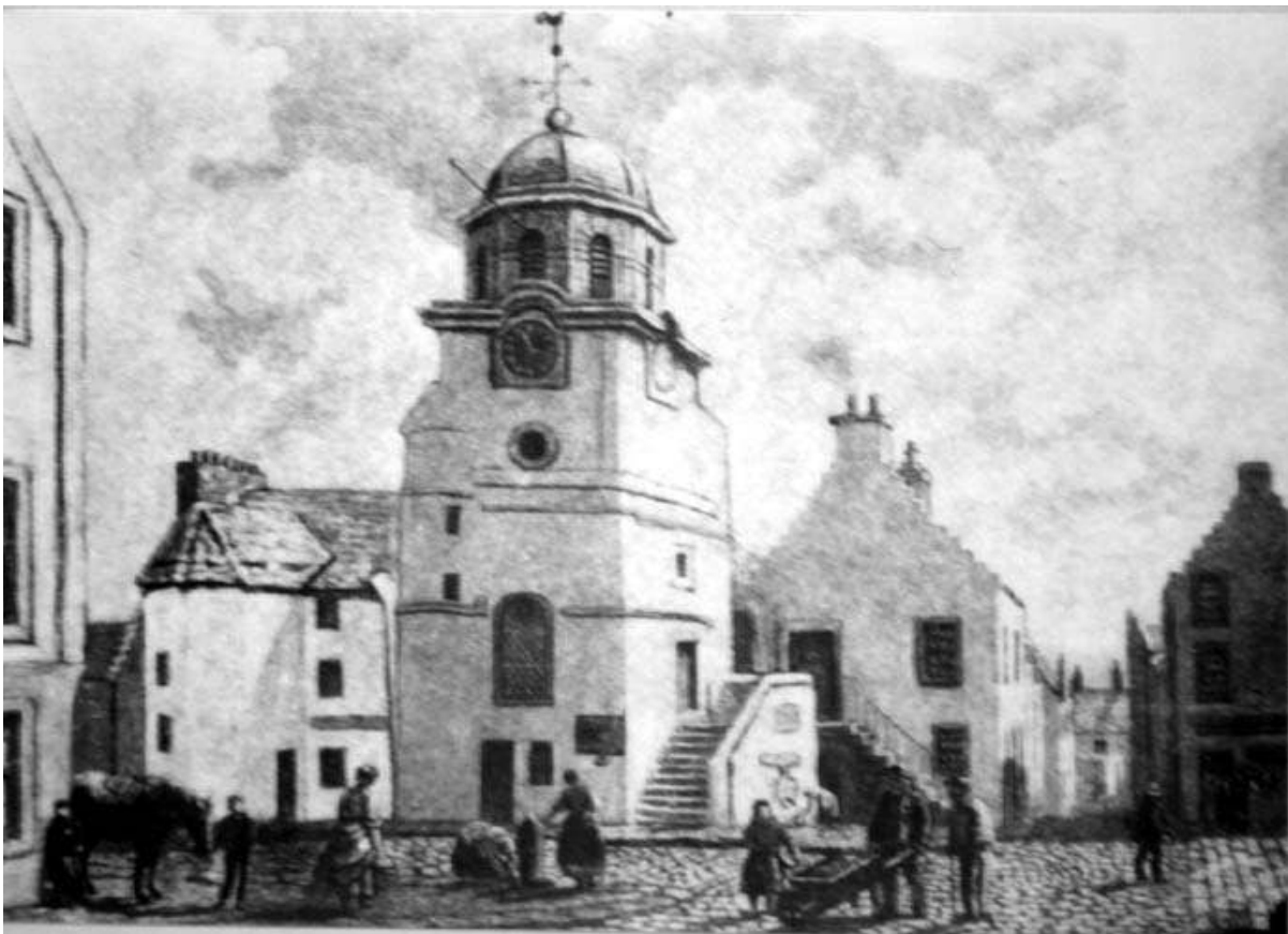
Fig 11: View, undated. This image suggests that the string courses and stair tower roof were originally limewashed. It also indicates two carvings on the forestair. It also shows clearly the end arched window.
