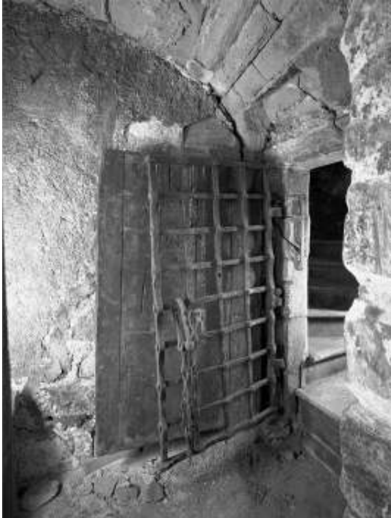
Fig 25: The Third Floor room.
