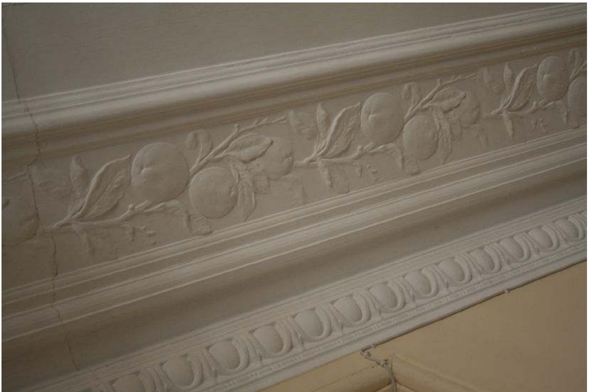
Fig 31: Detail of the cornice.
