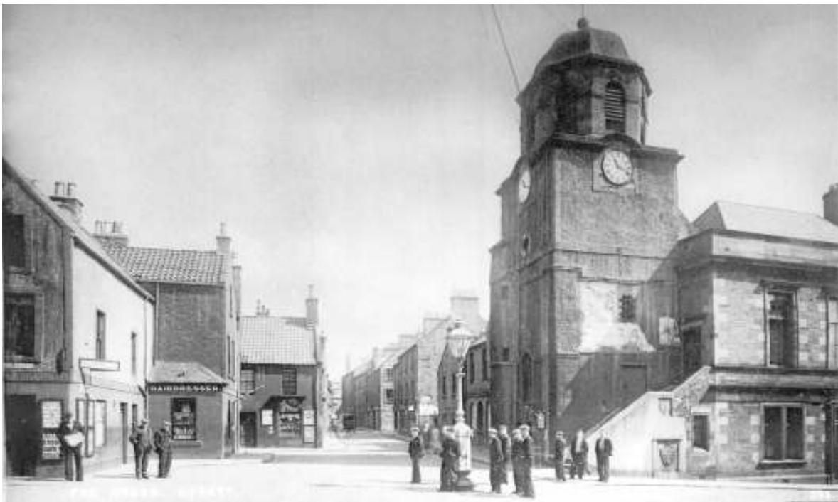
Fig 14: View undated. This photograph shows the flagpole and arched window, together with the two panels on the forestairs and the window that has since been blocked up.
